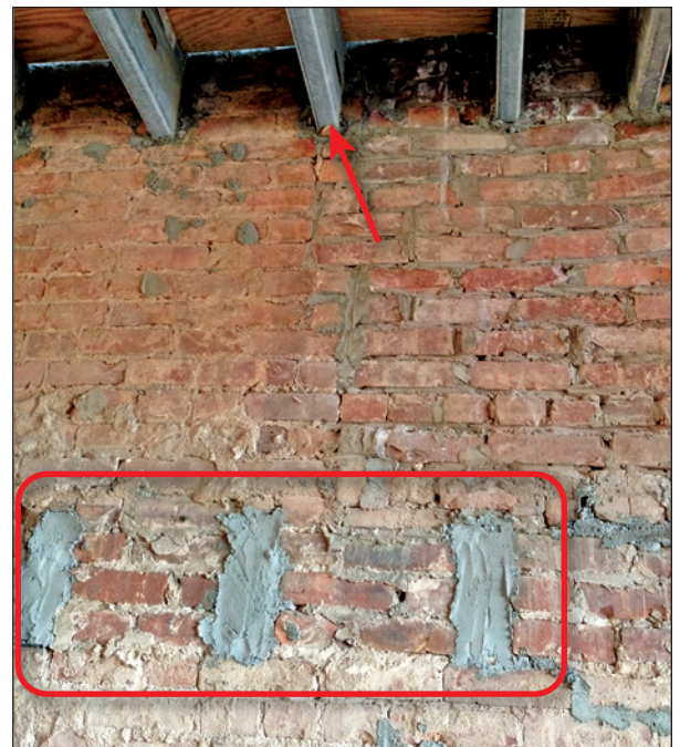
Figure 6: Elevation of a floor system in a row house. The old floor joist system (outlined in red) was removed and the gaps left by the joists filled. The new floor joist system (red arrow), designed by an engineer, was installed at a higher elevation (Brooklyn, NY).
