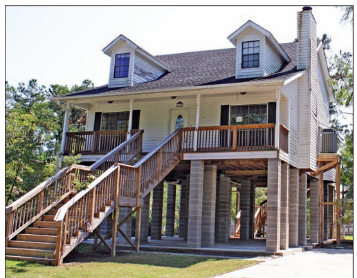
Figure 8: This house in Zone A was detached from its slab foundation (which remains) and elevated on masonry piers. The floor system is supported by new wood joists (Mandeville, LA).
