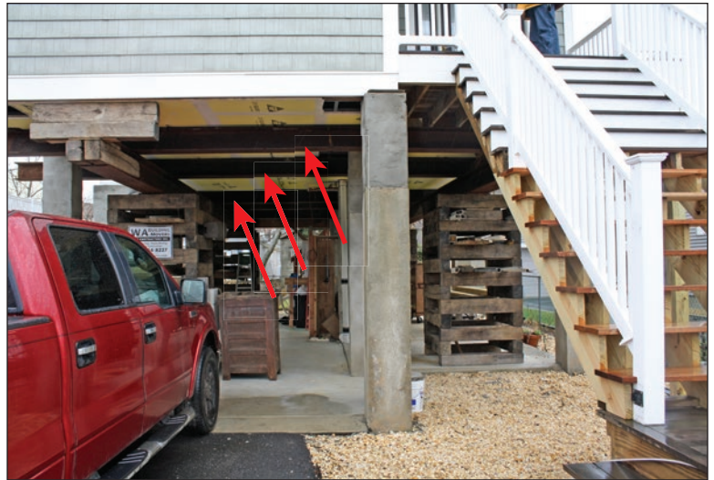
Figure 9: A house in the final process of being elevated in Zone A. The columns have been poured and the cribbing and steel lifting beams (red arrows) will be ready to be removed soon (Highlands, NJ).
